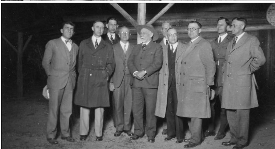
Photos on this page show the Tall Timbers camp in Recreation Park. At top is a view of the headquarters cabin constructed in 1925. The large field in front saw field meets, baseball games and various Scout competitions. The middle photo shows the construction of Troop 9's cabin within the eucalyptus grove. At bottom is the council Executive Board in front of the headquarters cabin sometime in 1927. The man in the hat at the center of the group is Daniel Carter Beard, one of the founding fathers of the BSA and its first National Commissioner. He was on a tour of western councils at the time. Scout Executive C. L. Appling is second from right.
